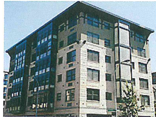
Cornerstone Condominiums SW Jefferson, Portland (46 units) Built 1999
